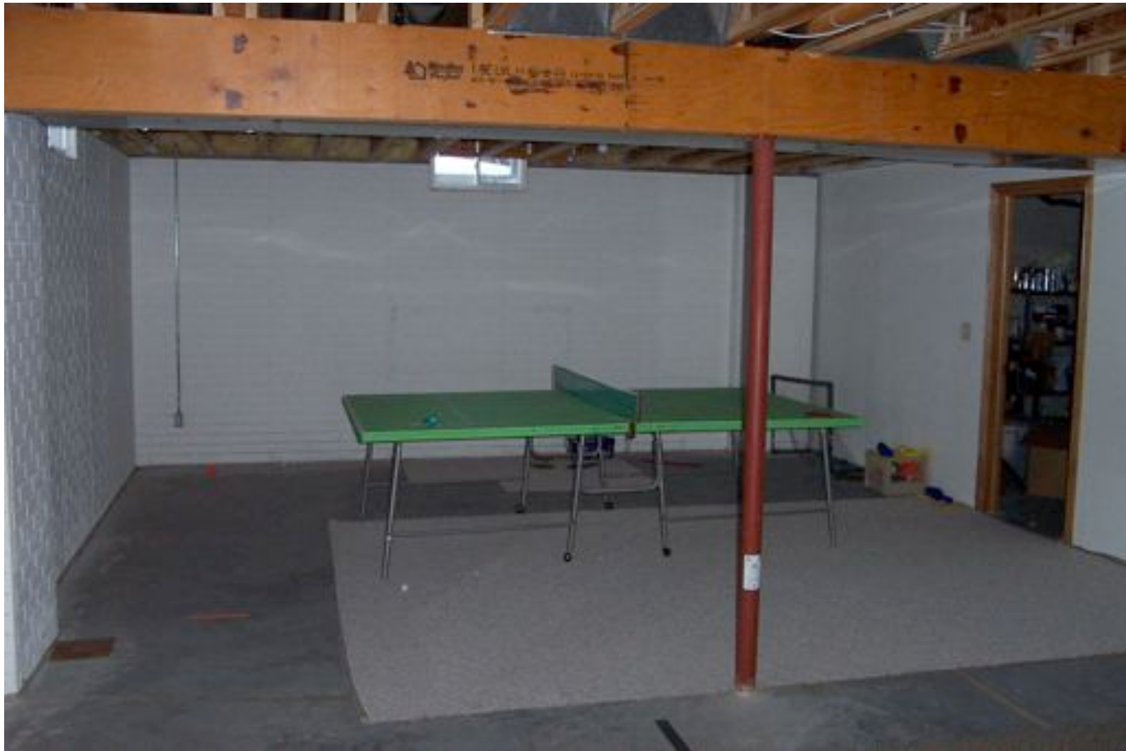
Partially finished basement
