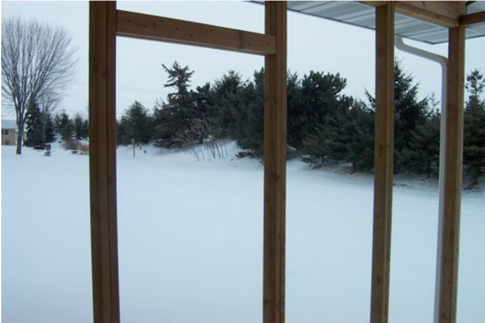
Left backyard view from dining area thru unfinished screen porch
